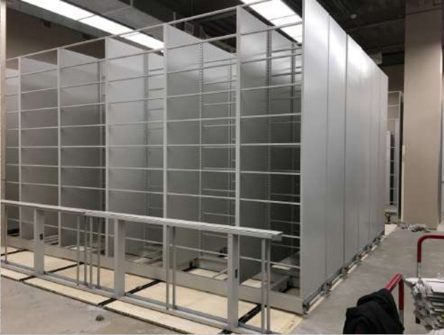
New compact shelving units, custom sized and designed to maximize space in the CPM's archival storage room and increase accessibility of the Center's valuable materials.
