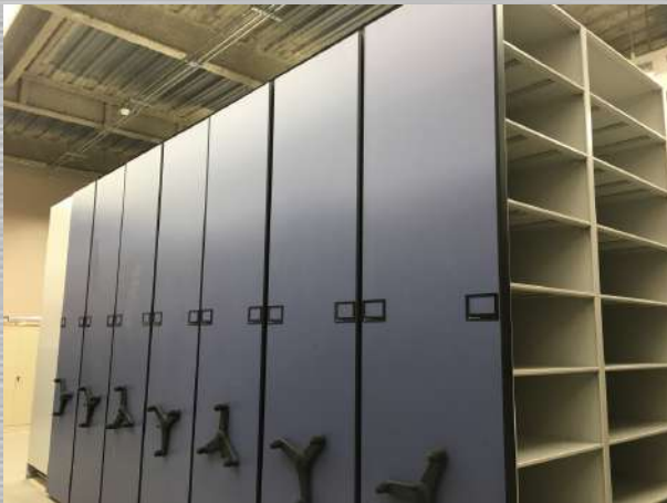
End panels (in MTSU Blue!) installed, along with geared handles to move the new shelves with ease.
